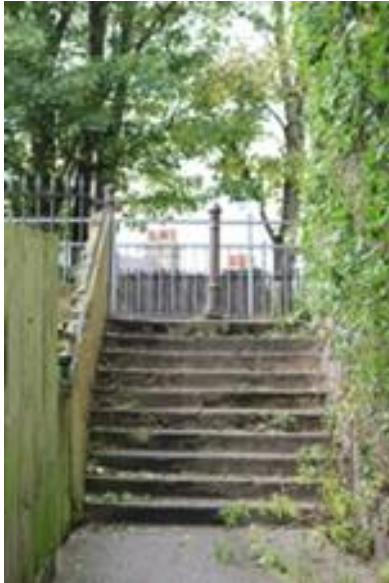
Boundary Post from passageway
