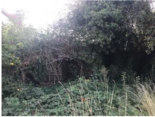
Outside of east wall bordering amenity green
