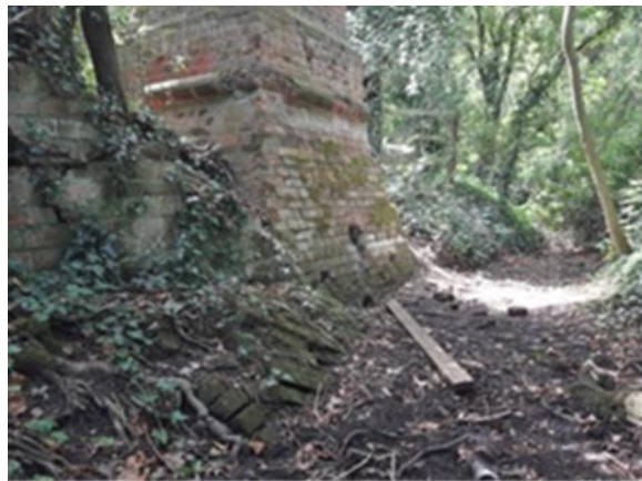
Base of Stench Pipe from channel showing brick revetment
