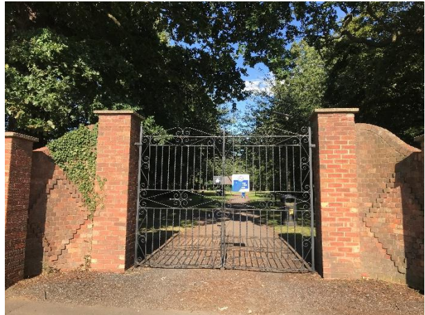
Original wrought iron gates, Dilkes Park 2020
