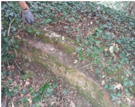
Brick edge to circular structure
