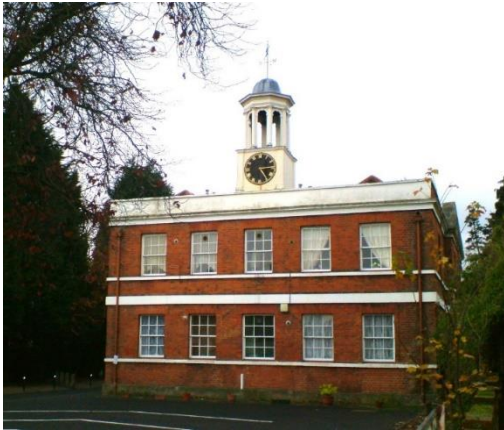
The Clockhouse Building 2004
