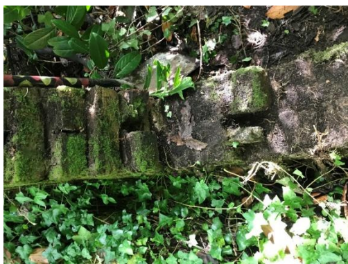
The Pump House. South wall detail of brickwork showing recesses for perhaps a metal grating?
