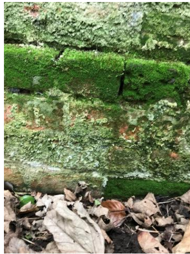
Moss covered plinth of rear of garden wall
