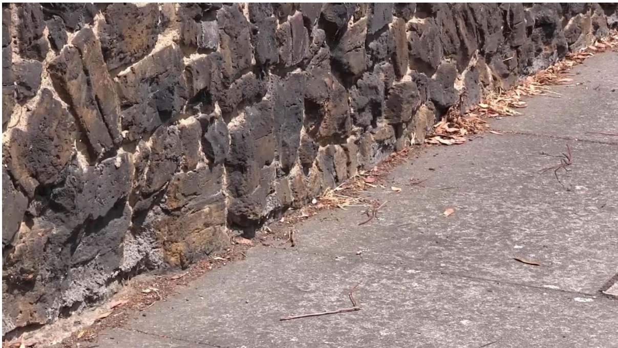
"Reject Brick" Wall – Herbert E. Brooks Memorial Rest Garden
