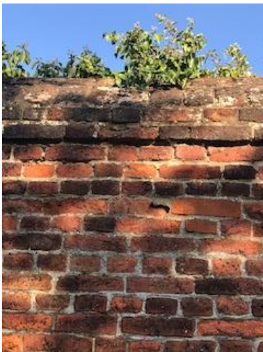
Wall showing English Bond and gabled capping
