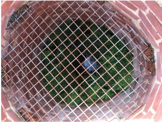
Interior of Walled Garden Well showing both modern and older brickwork
