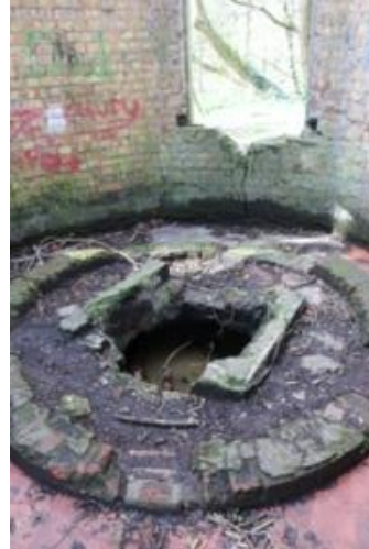
Well head inner chamber
