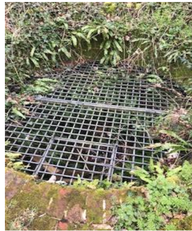
Padlocked metal grid covering the icehouse well
