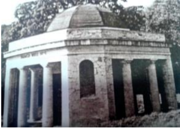
Pump House nineteenth c1924
