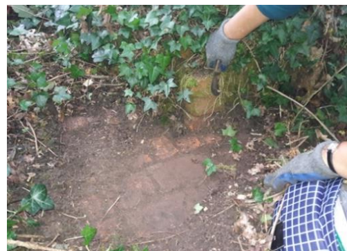
Brick floor showing edge of culvert
