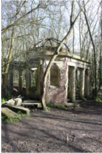
Pump House from the south
