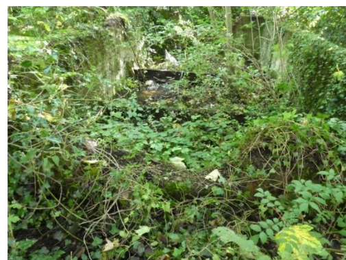
The Pump House looking N-S showing broken walls at the north end. The girders can be seen through the debris and bramble
