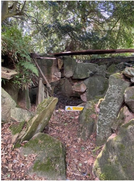
Gorge entrance to Filmy Fern Cave showing remains of timber entrance gate, stone arch with keystone and steel roof supports
