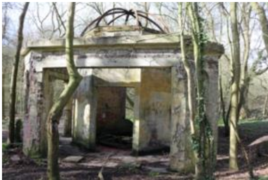
Pump House from the east
