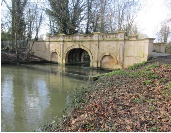
Parklands Bridge post- restoration 2020
