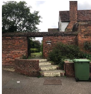
Side entrance to garden in west wall
