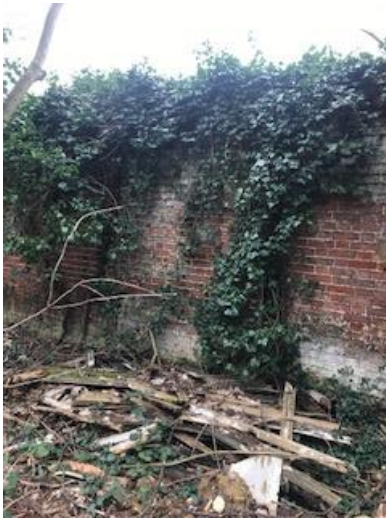
Rear of wall overgrown with ivy and scattered fly tipping, 2020
