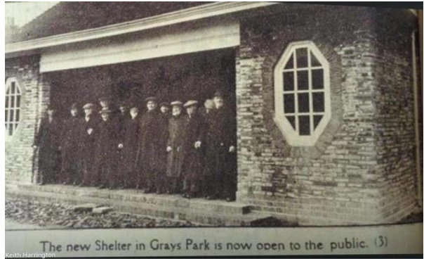
Grays Town Park Shelter c1930
