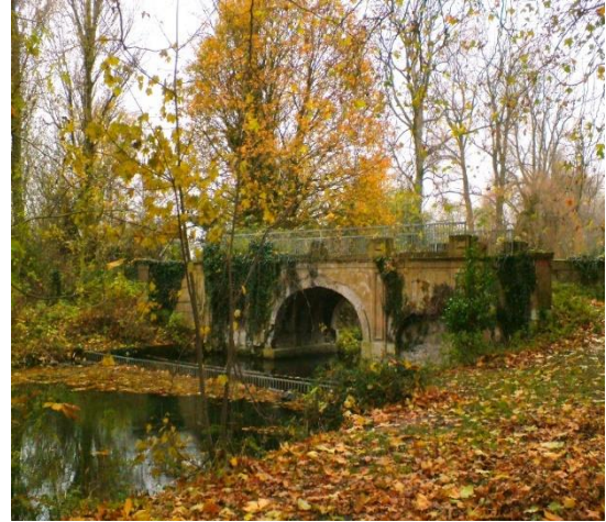
Parklands Bridge pre-restoration
