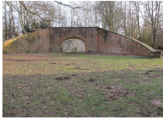
Retaining brick base of Belvedere Tower 2020
