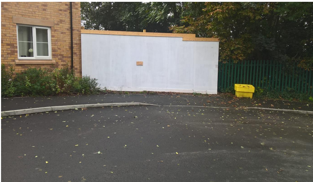
Railings to the right of the (now boarded) access to viewing platform
