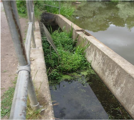
Sluice and dam at south end of pond 2020
