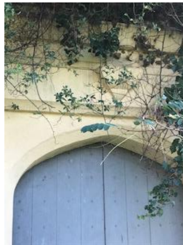
Gated entrance to north wall showing cornice
