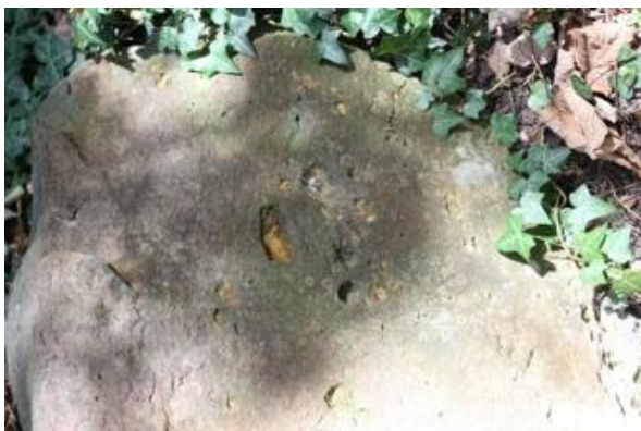
Closeup of rock with possible brick core showing through outer layer
