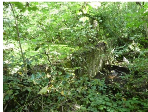
The Pump House showing the building and proximity of the large water reservoir (thick with duck weed)
